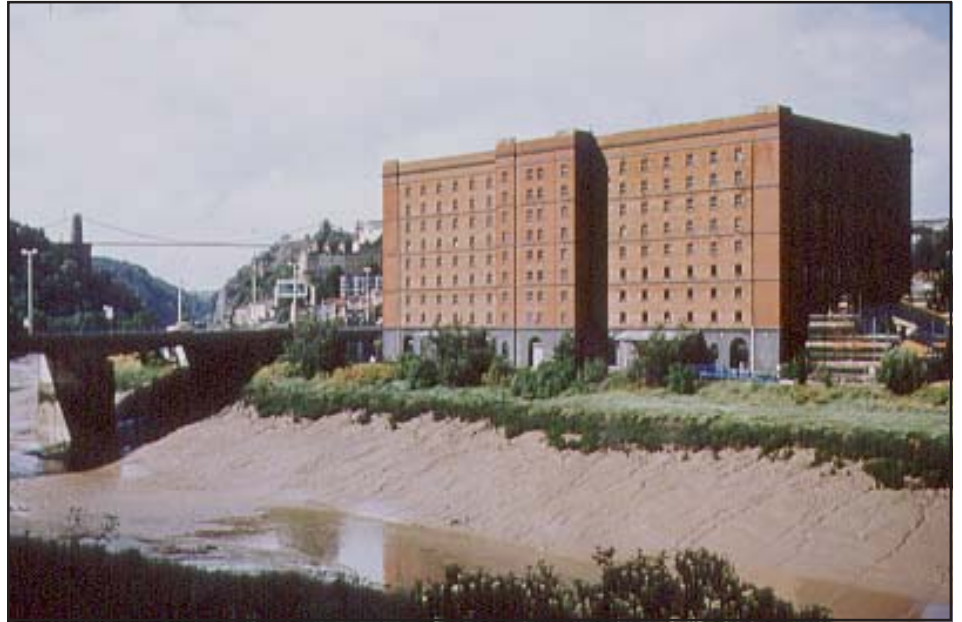
"B" Bond Warehouse, home of the Bristol Record Office
